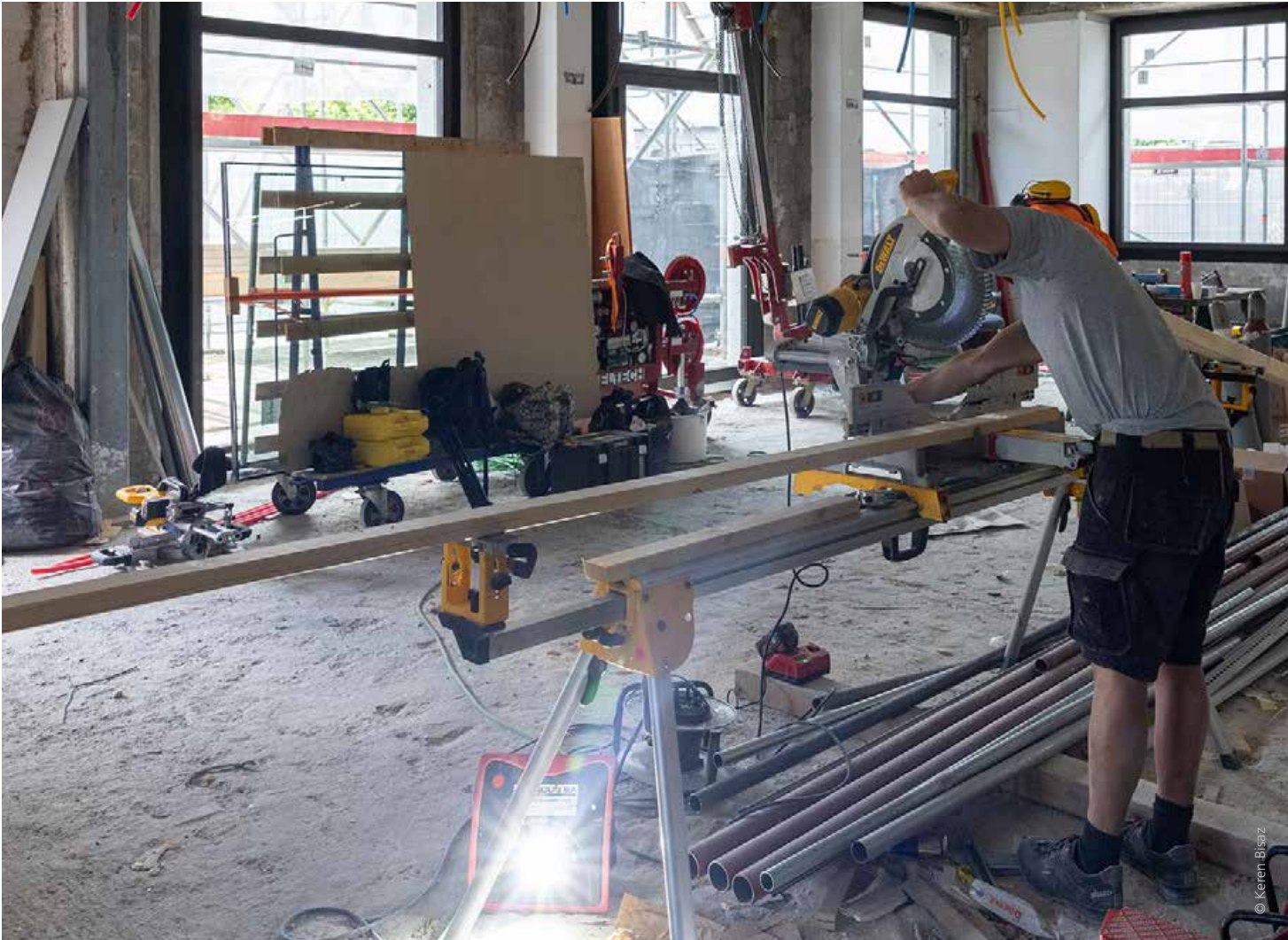
Renovation of the Bulle branch, Place du Tilleul
